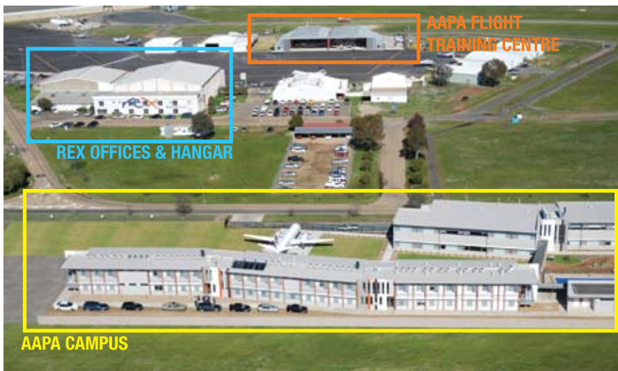
Aerial view showing the proximity of the AAPA Campus to the AAPA Hangar (also the Flight Training Centre), and to the Rex Offices and Hangar
